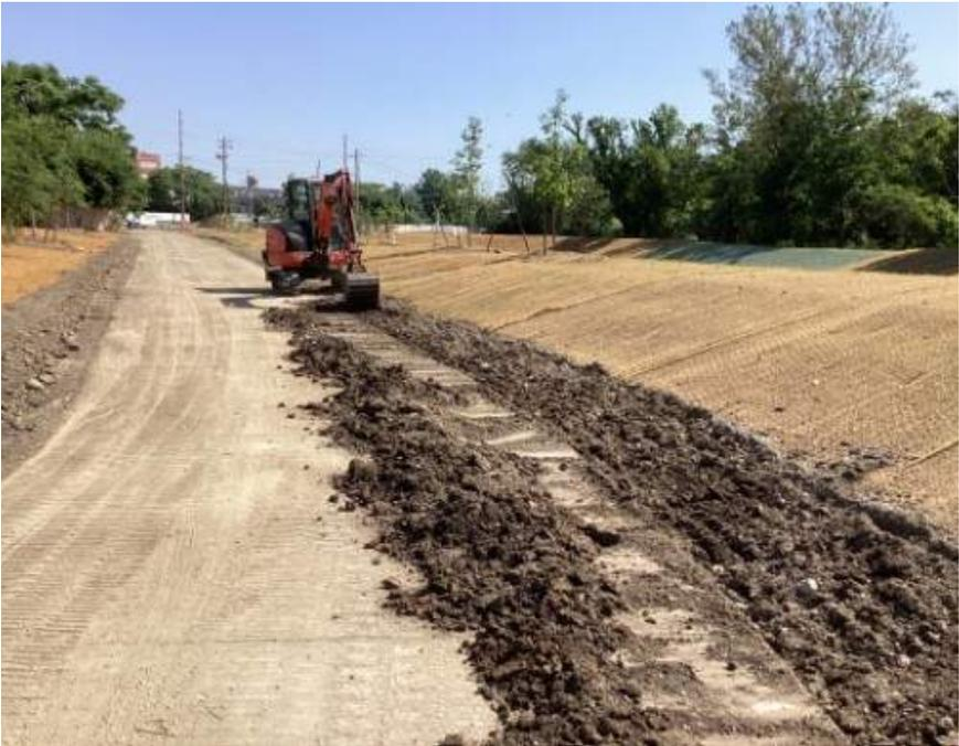
Phase II excavation and subgrade preparation for sod installation adjacent to the multi-use trail near the east flood storage basin.
