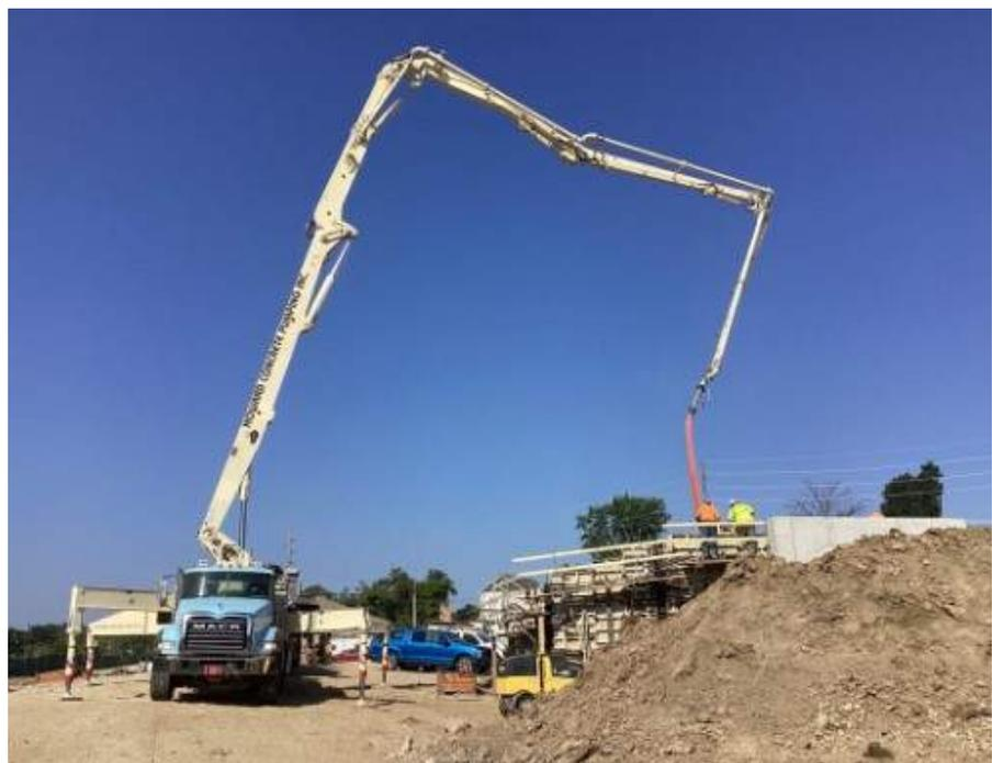
Destination Playground concrete pumping for the cast-in-place retaining wall.
