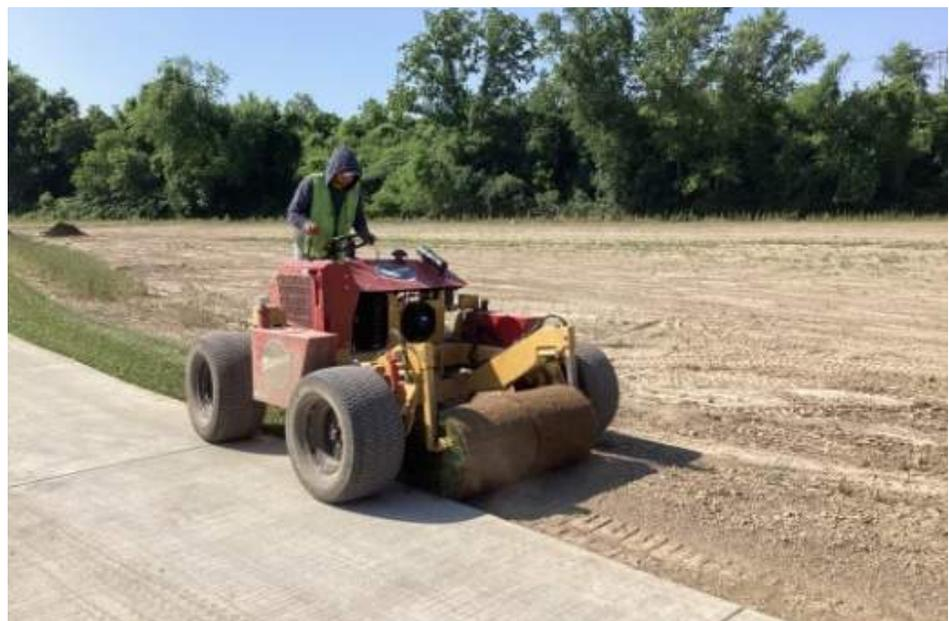
Phase I sod installation adjacent to the multi-use trail in the low-lying area within the floodway.
