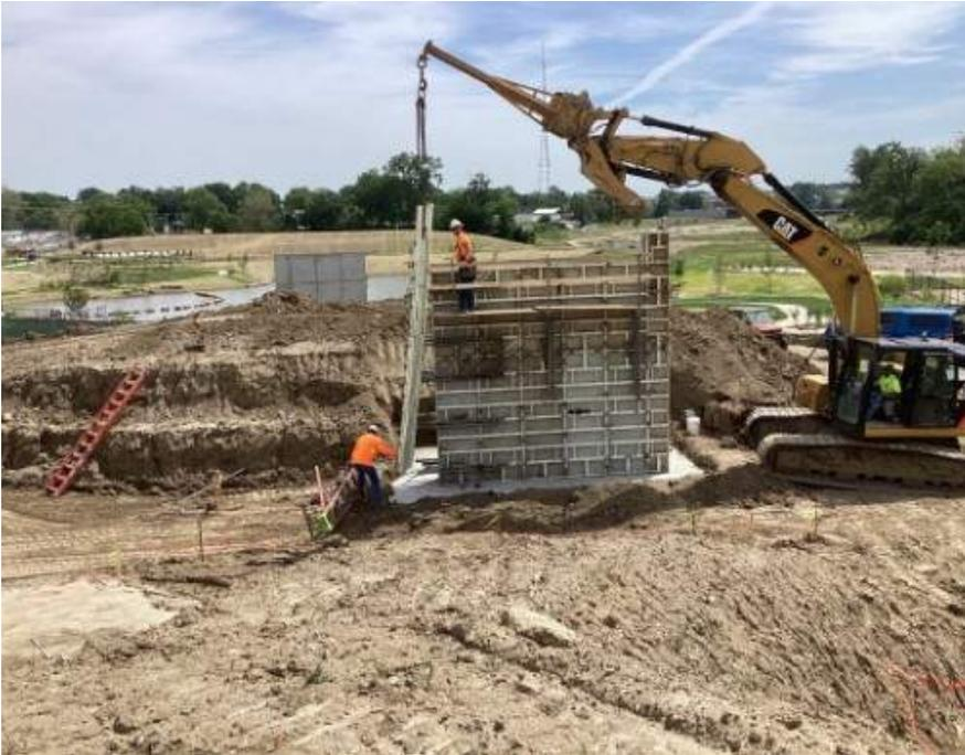
Destination Playground cast-in-place concrete retaining wall formwork installation.
