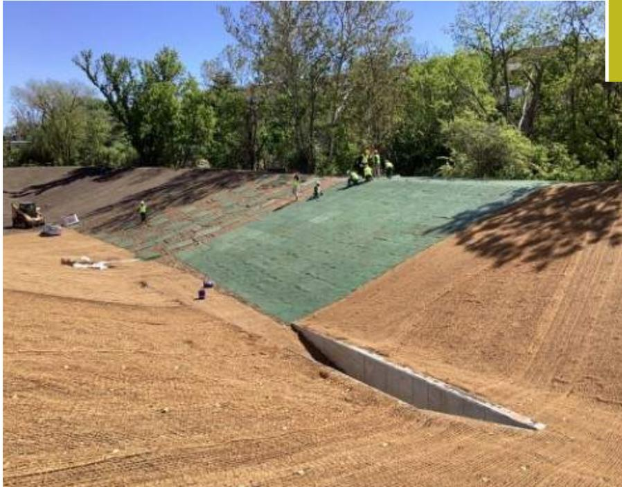
Phase II revetment protection mat installation at the overtopping weir at the east flood storage basin.
