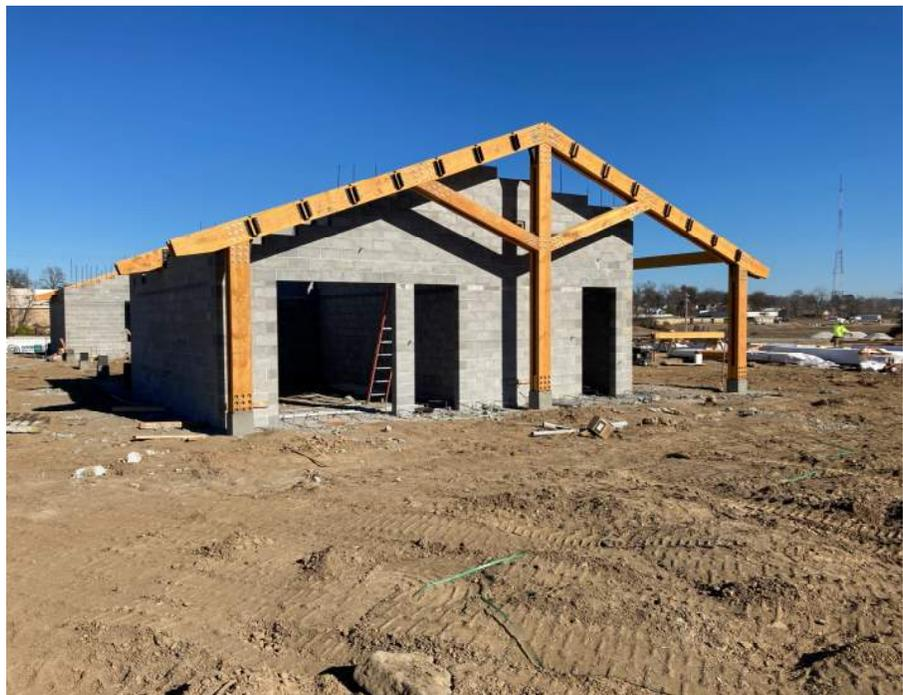
Comfort Station Event Room area masonry construction and timber framing.
