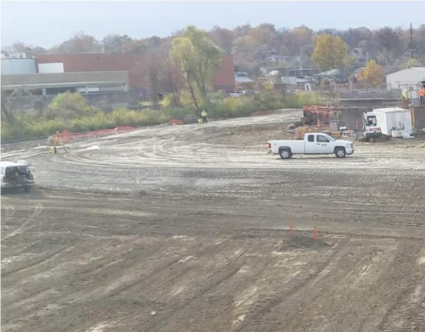
GRG Connector Part A construction staking and layout for new storm sewers.
