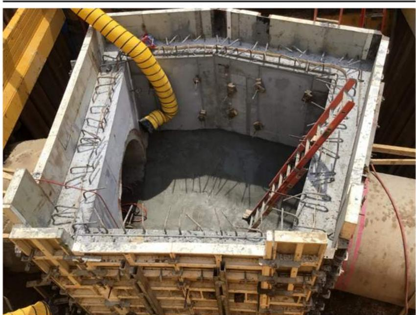
Downstream junction chamber for tie-in of the new 72" sewer line and the existing horseshoe sewer.
