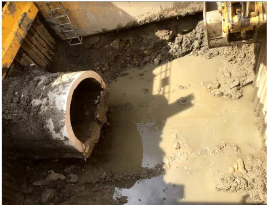
Excavated pit for construction of the upstream junction chamber and tie-in of the new 72" sewer line.
