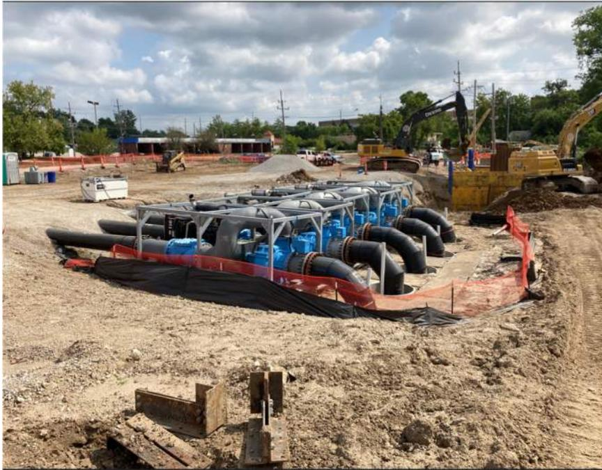
Downstream bypass pumping operation and construction of the downstream junction chamber.
