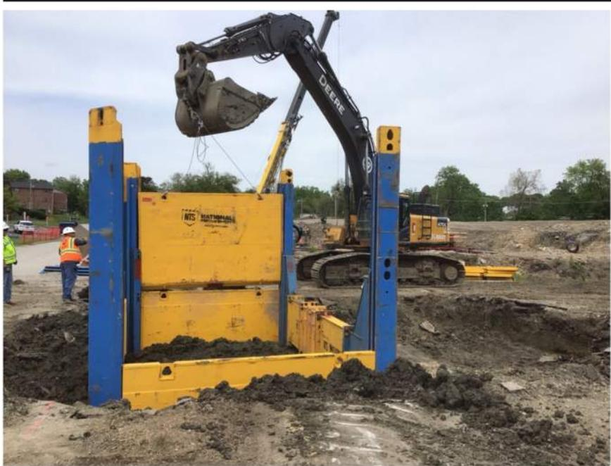
Slide rail shoring system installation for the large sewer junction chamber at Mary Avenue.
