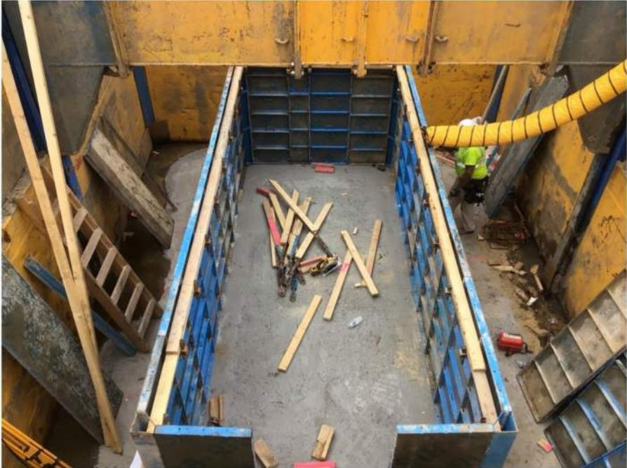
Formwork installation for the large sewer overflow structure at Mary Avenue.
