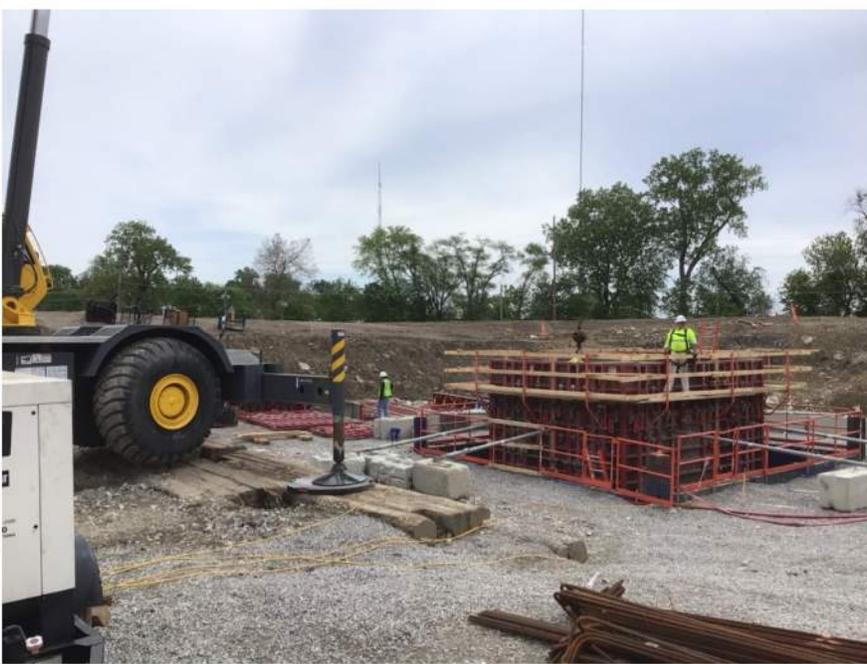
Formwork removal for the large sewer overflow structure at Mary Ave.
