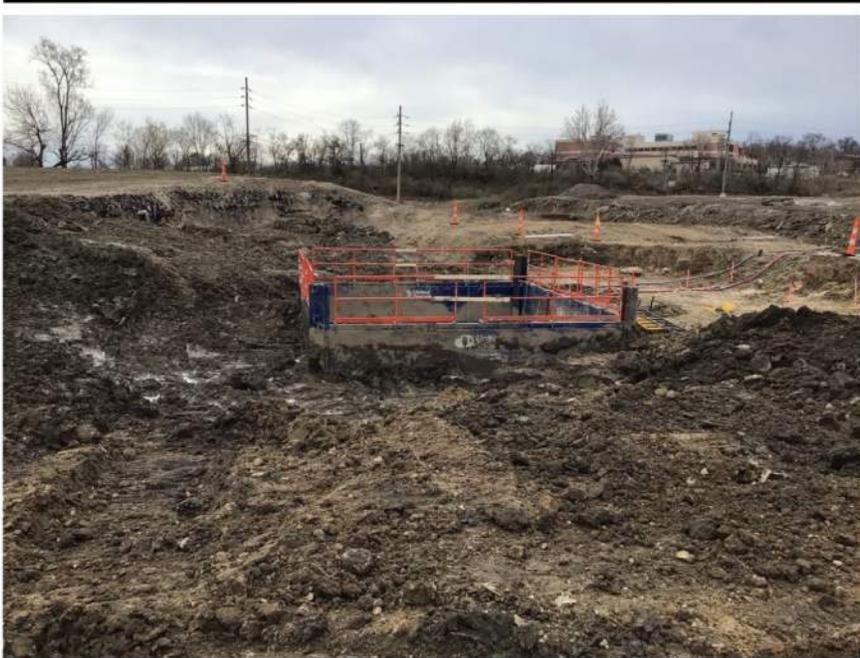
Shoring box system and safety railing for the large sewer overflow structure at Mary Avenue.
