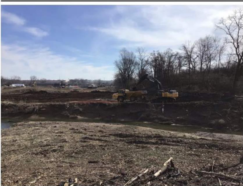
Mass excavation, material loading, and excavated material haul-off operations at Parcel #93.
