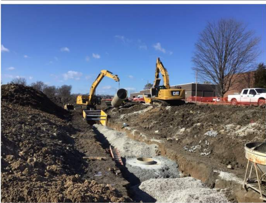
72" sewer installation along Brentwood Industrial Ct.
