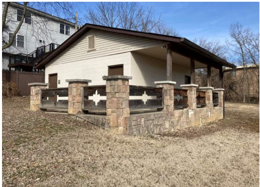
Norm West Park restroom facility scheduled for demolition under Demolition Package 1C.
