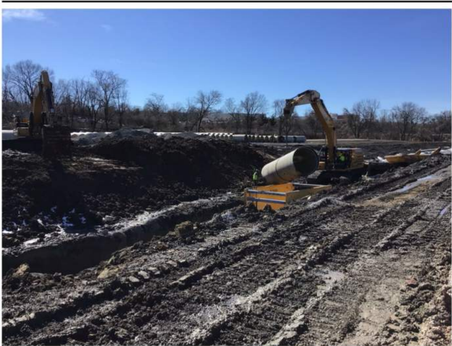
72" sewer installation along Brentwood Industrial Ct.
