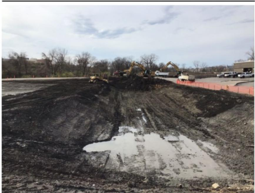
Photo of mass excavation work for the benched down area for the proposed 72" FRP pipeline. Photo taken at alley between building sites #77 and #78 looking West.
