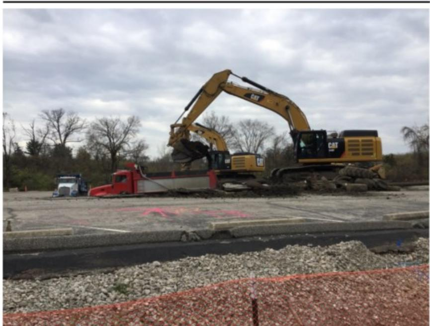
Loading of the tandem dump trucks for the mass excavation on Parcel 77.
