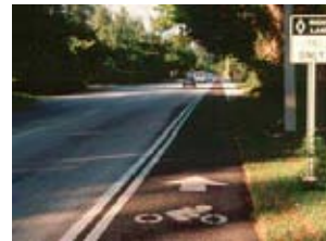
30. Bicycle lane treatment.
